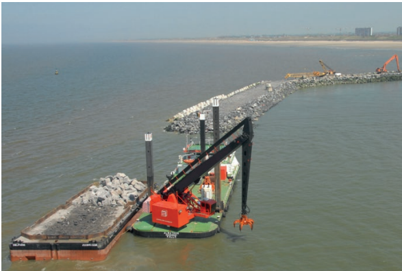
Crane vessel / Rock installation
